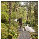
Sept 28: It was all hands on deck out at Point Bridget the past few weeks! To improve the trail, we first removed a ton of old, slippery boardwalk. Much of this boardwalk was rotting away or falling into puddles on the trail. Once the boardwalk was out, crews began to add gravel to the trail.
