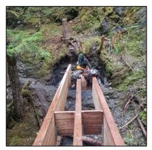
largest on Treadwell Ditch (only 4 feet shy of Lawson Creek for those curious). It required excavating rock in order to create space for one of the bridge's abutments, building gabion baskets for the abutments, flying in bridge beams that weigh 2200 pounds, and harnessing up in order to install beam braces and decking.
