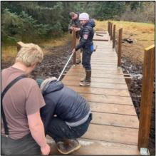
Getting this right was important to facilitate easy access to SAIL's ropes course, as some participants may have different mobility needs. The new walkway is also higher than before to ensure the structure will be above typical flood waters, which should make it safer as well as last longer.
