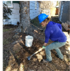
SHOVELING -Use a grubbing tool to decompact material before moving it with a shovel -Avoid twisting and extending the shovel far from your core -Step towards your offloading site rather than flinging materials long distances
